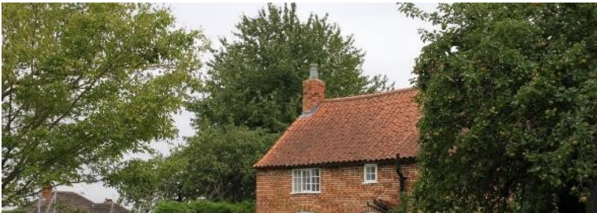
Traditional Welsh Slate and red pantile ROOFS
